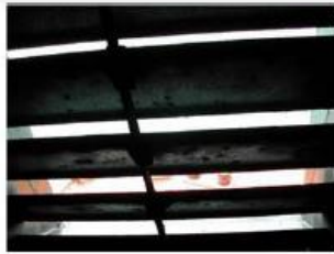
Fire flaps unable to close tight
