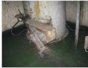
Hydraulic operated closing device not in good working condition
